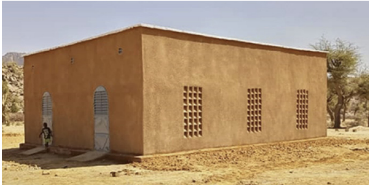
Onion Storage Barn, Mali (Source: AVN)
